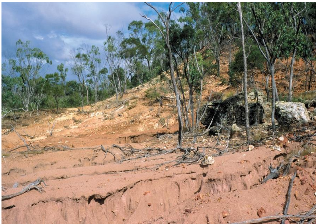
Fig 5: Sheet and Gully Erosion
